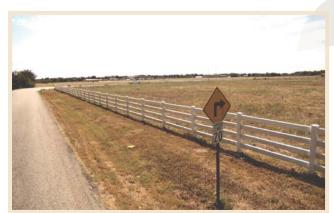
The sign above represents typical "Fair" sign conditions. The sign is slightly tilted and faded, but is still clearly legible.
